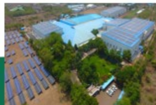
Solar Panels at Pune mill, India
